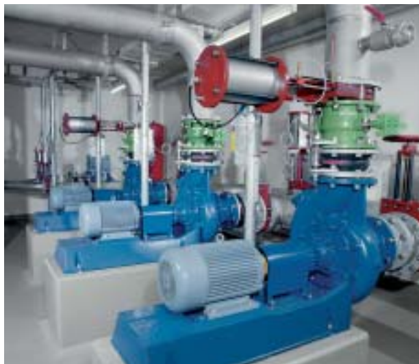
Process pumps installed horizontally on a base-plate for fast service.
